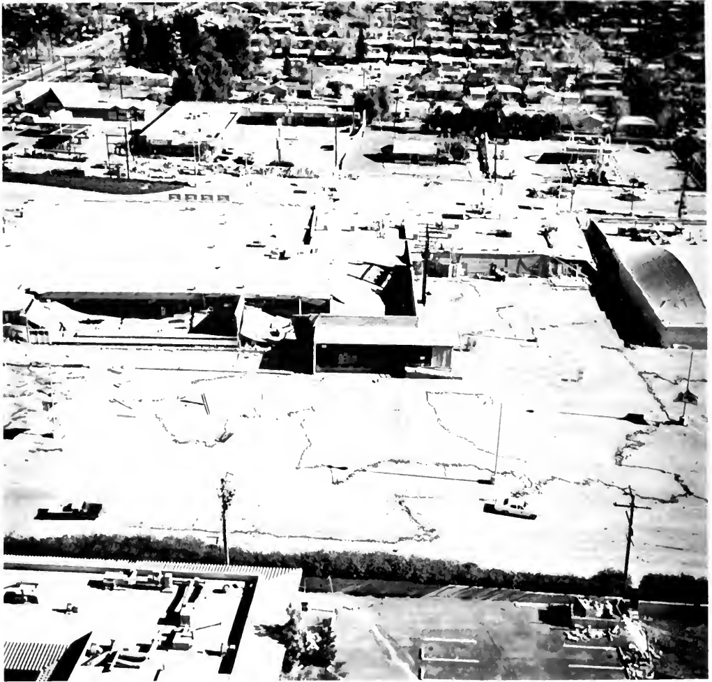
Photo 5. Boys Market, at the corner of Glenoaks Boulevard and Hubbard Street, collapsed as a result of ground displacement and ground lurching in combination with intense shaking. Photo courtesy of Robert E. Wolloce, U.S. Geological Survey.
